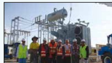
Erected Transformer in AUS.
