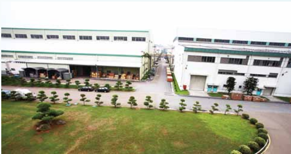
Heavy Electric Plant's picture (inside view)
