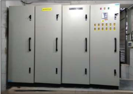
2400 KVAR APFC Grameenphone Switch at Nobinogor, Savar
