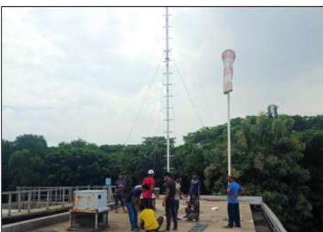
LPS, OPR-60 Saidabad Water Treatment Plant
