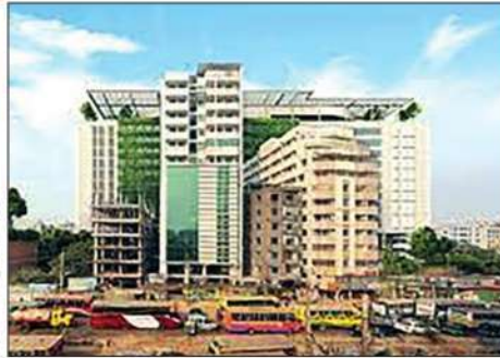
ABB Switch & Socket BRAC University - New Campus
