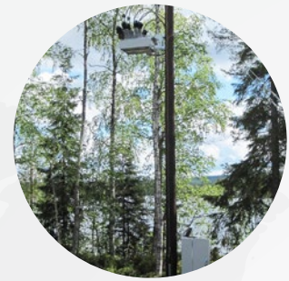
UNDERGROUND TO OVERHEAD CONNECTION
